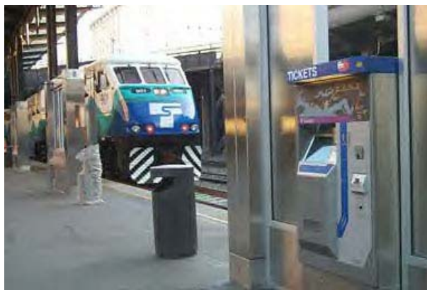
Figure 9.9 Ticketing at Vending Machines on the Platform
