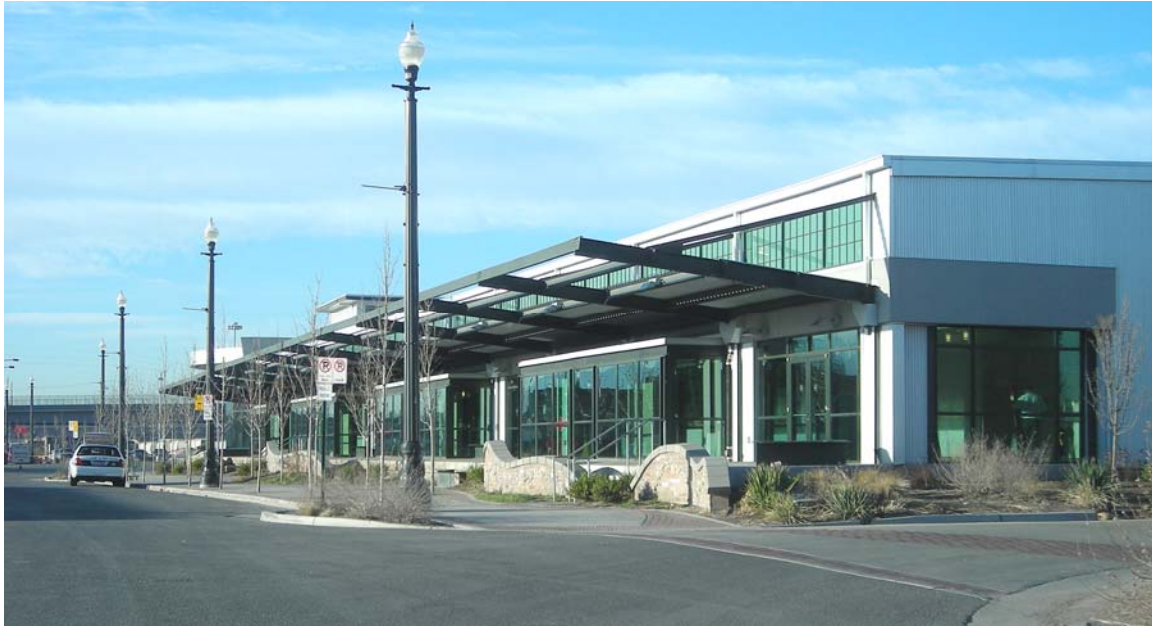
(above) Looking south toward the Hub entrance. The northern half of the Hub building houses the Greyhound Bus terminal and offices.
