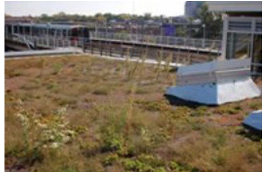
The Bethel New Life Center is a "green" building, featuring photovoltaic cells to make the building more energy self-sufficient, recycled materials, and a living rooftop garden. (Photo: Graham Garfield, www.Chicago-L.org )
