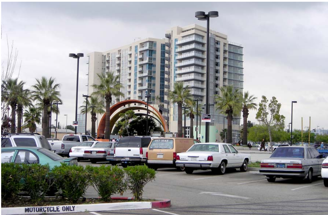
New housing at the park-and-ride for the North Hollywood Red Line station.
