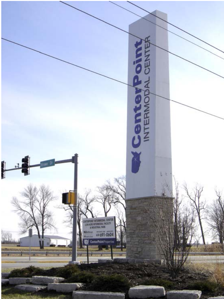
CenterPoint Intermodal Center near Joliet, IL, brings together rail and highway freight movement, with nearby links with waterborne freight movement.
