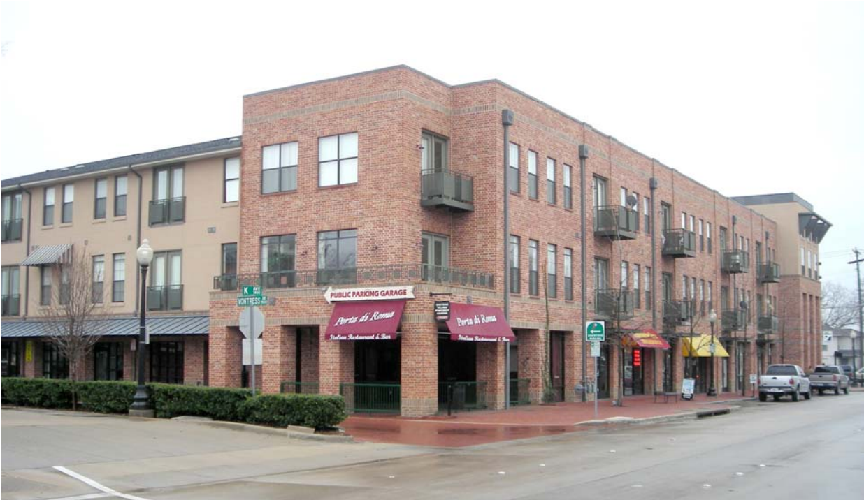
New, medium-density housing in downtown Plano near the Downtown Plano DART station.
