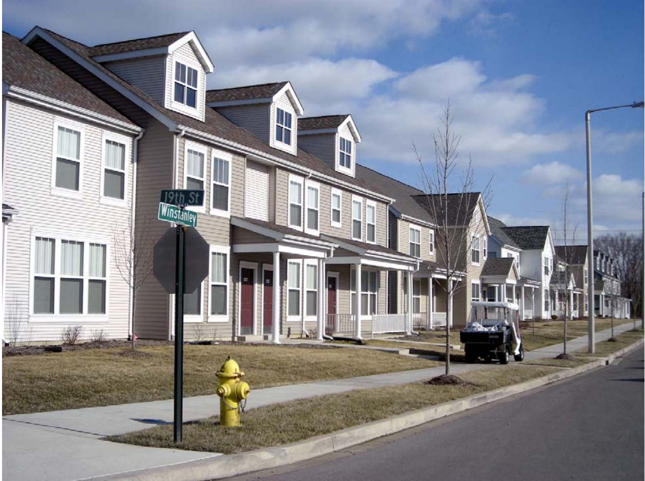
New townhouses in Emerson Park, about one block from the station, across the street from the Community Center building.
