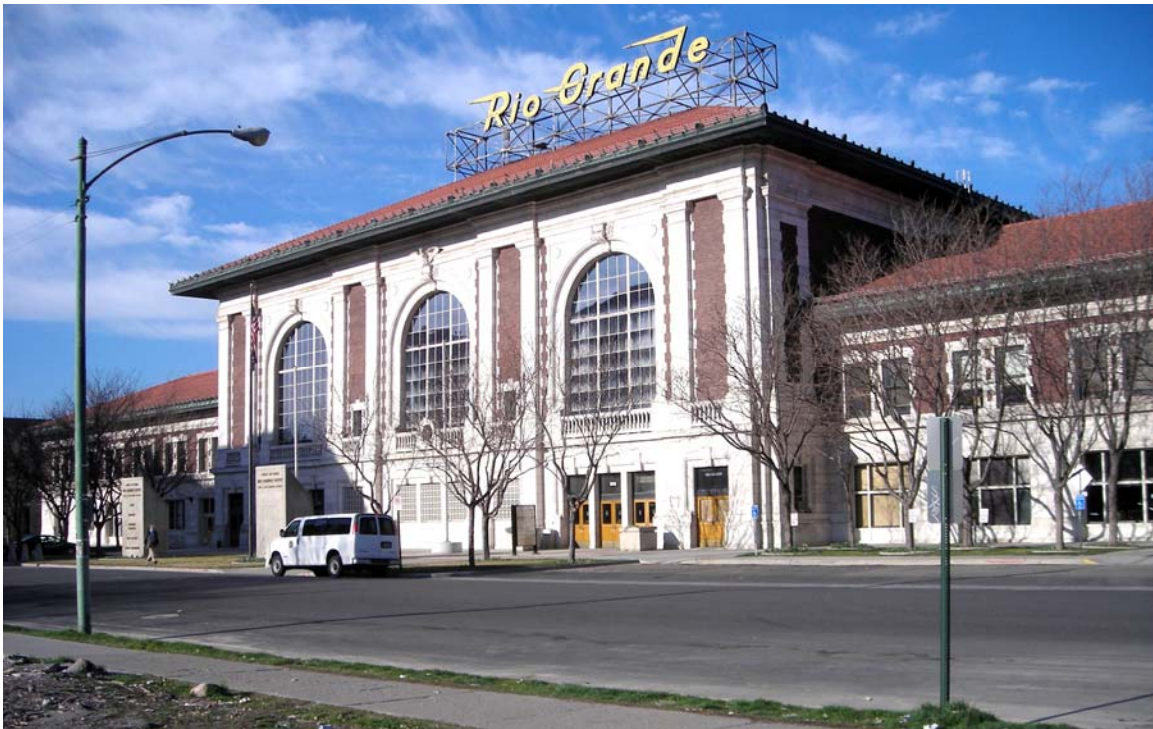
(below) Between the Hub and the downtown center, the old Rio Grande railroad station now houses a historical museum.
