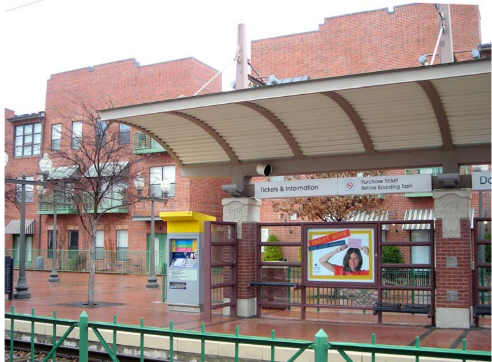
New housing and ground-floor commercial activity adjacent to DART's Downtown Plano Station on the Red Line.
