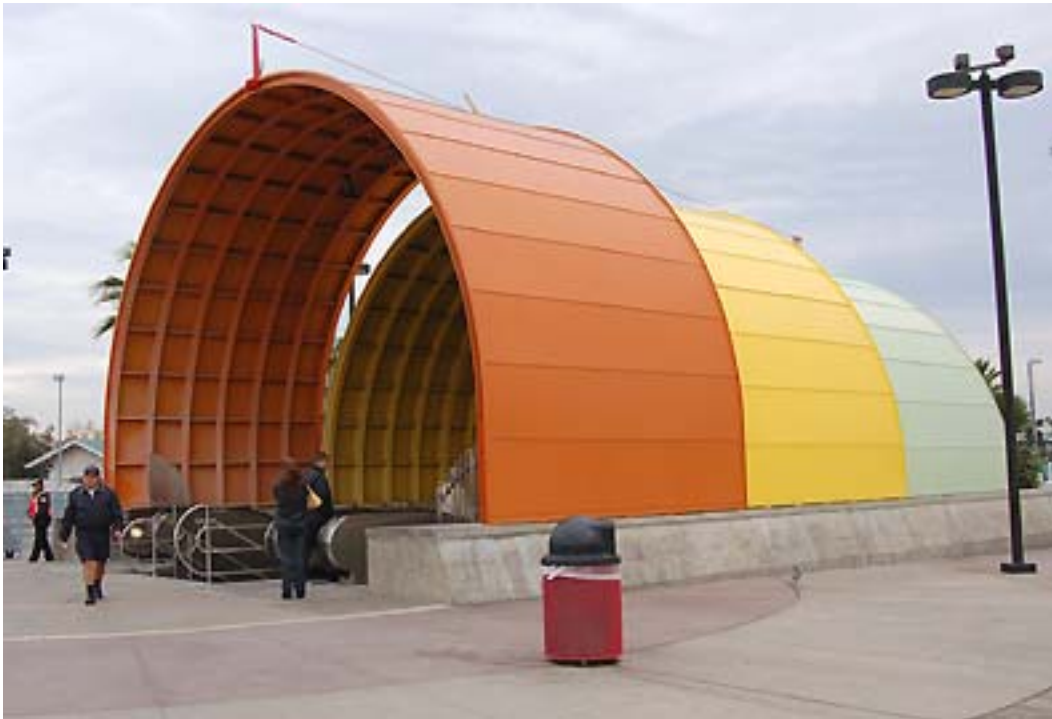
Entrance to the North Hollywood Red Line METRO station. (Photo: Jim Horne, West Coast TNDs)
