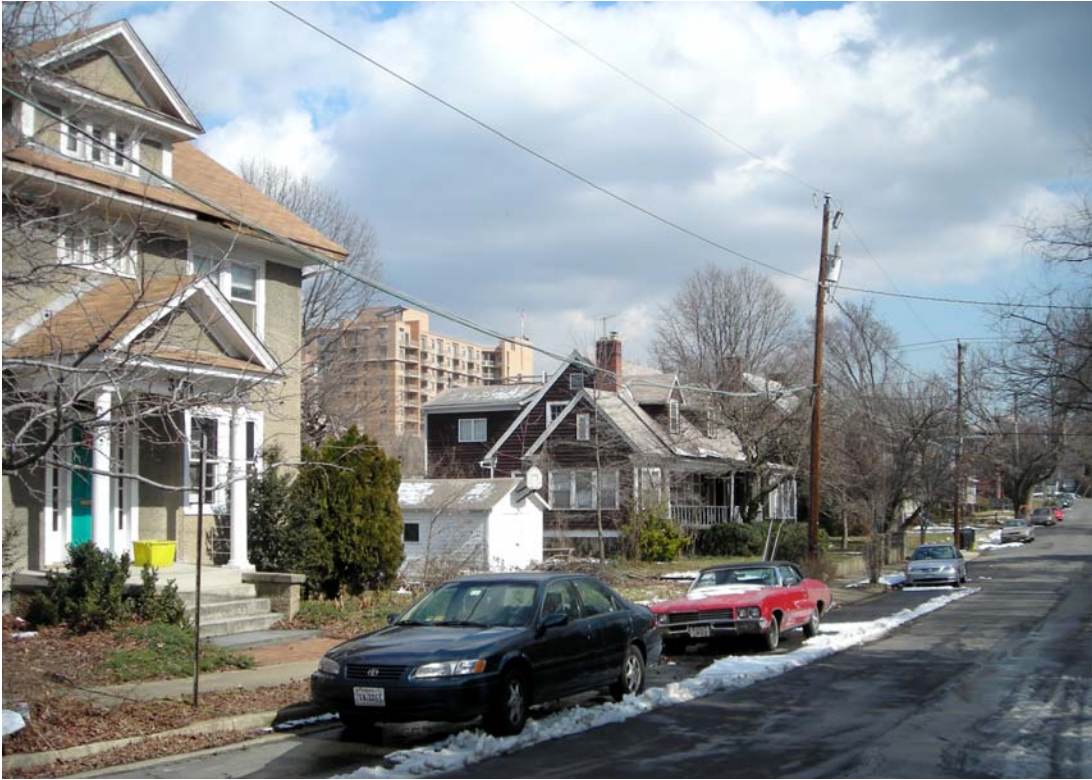
(above) A 1920s-era neighborhood near the Clarendon METRO station in Arlington, protected from pressure for high-density development close to the METRO (background).
