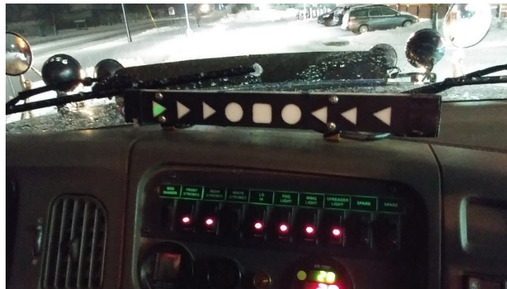
Figure 6.1. Image of the lane boundary guidance system mounted in a MnDOT snow plow truck.
