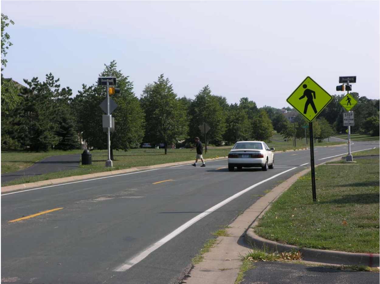
Figure B-15. Site 15 (see table above). Pedestrian-actuated warning crosswalk in Woodbury across Interlachen Parkway, looking south.
