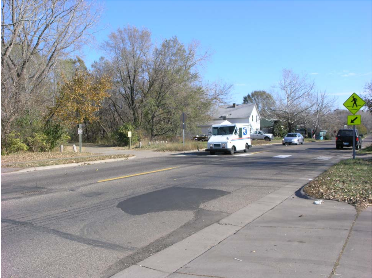
Figure B-3. Site 3 (see table above). Passive warning Gateway State Trail crosswalk in St. Paul across Arlington Ave., looking west.
