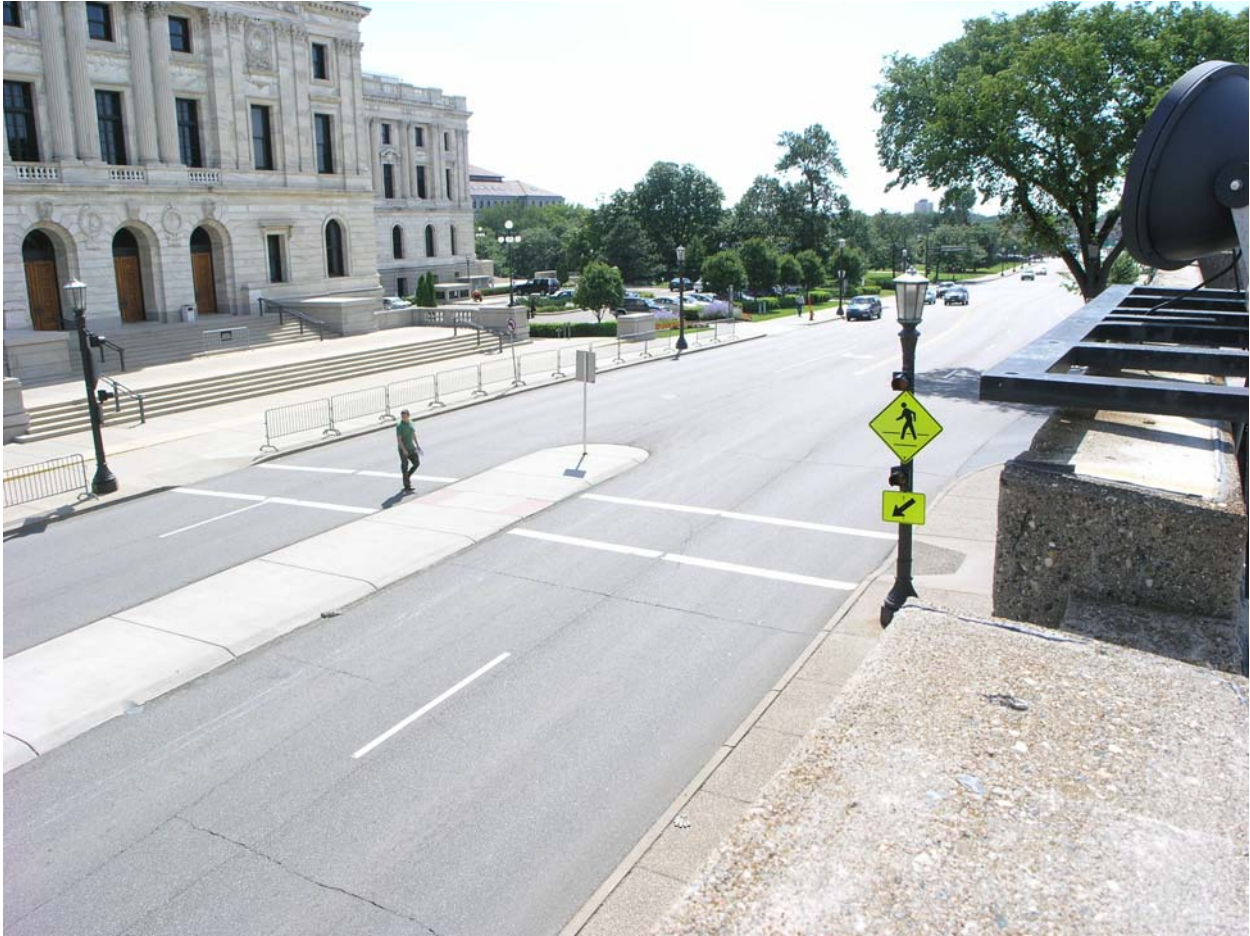
Figure B-11. Site 11 (see table above). Continuously active warning crosswalk in St. Paul across University Ave., looking west.
