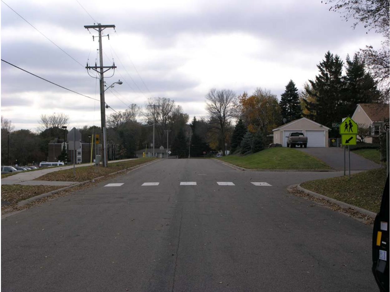
Figure B-6. Site 6 (see table above). Passive warning crosswalk in Roseville across County Road B, looking east.
