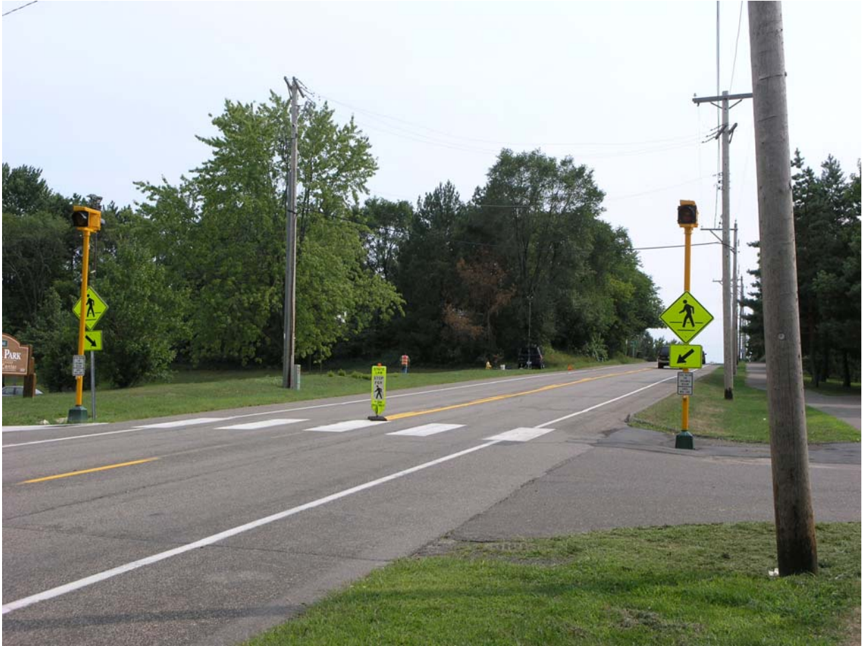
Figure B-18. Site 18 (see table above). Pedestrian-actuated warning crosswalk in Roseville across Dale St., looking south.
