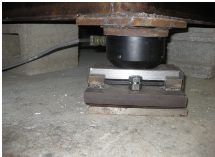
Figure C-3: Load cell installed under device
