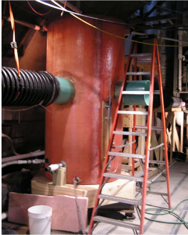
Figure 2.1. 4×4ft Sump and Test Stand
