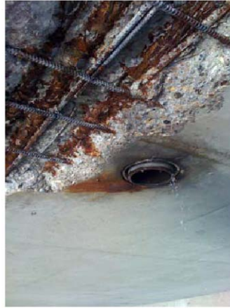
Figure 6.4. Bottom slab drainage outlet (Corven Engineering, 2010)
