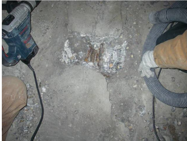
Figure 6.31. Removal of concrete exposing tendon B28
