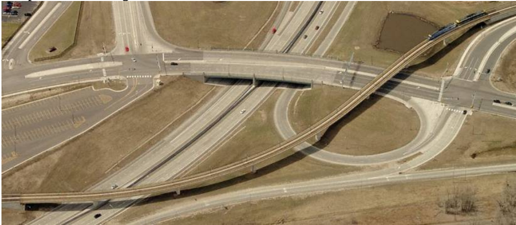
Figure 4.5. Bridge 27262 aerial view (Bing, 2011)
