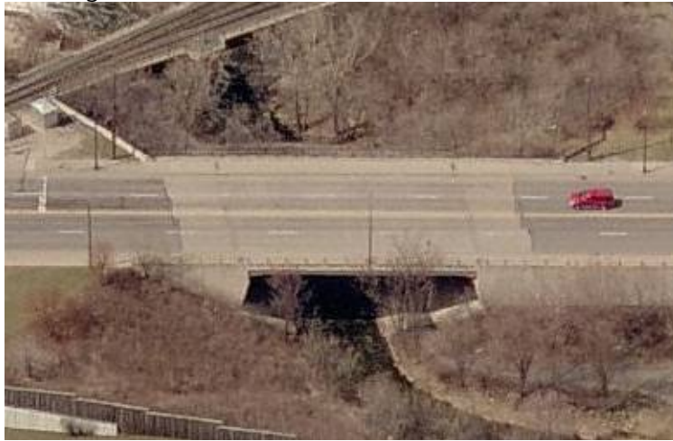
Figure 4.15. Bridge 27719 aerial view (Bing, 2011)
