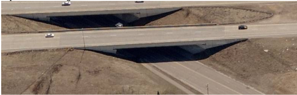
Figure 4.39. Bridge 70038 aerial view (Bing, 2011)
