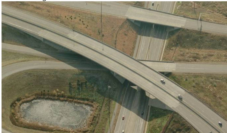
Figure 4.8. Bridge 02037 E aerial view (Bing, 2011)
