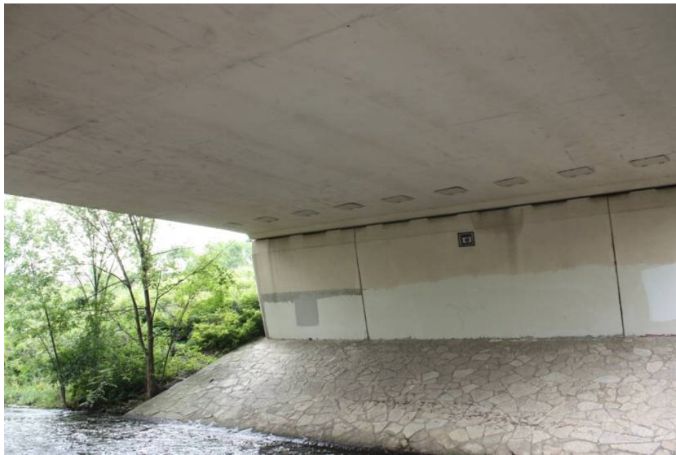
Figure 5.7. Bridge 27719 overview picture
