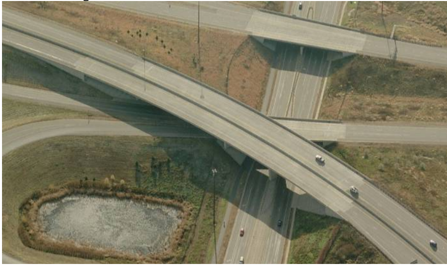
Figure 4.11. Bridge 02037 W aerial view (Bing, 2011)
