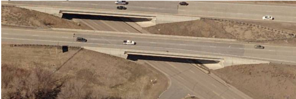
Figure 4.34. Bridge 70037 aerial view (Bing, 2011)
