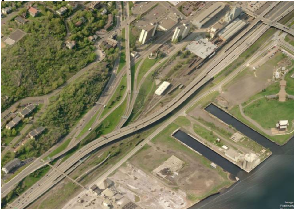
Figure 4.28. Bridge 69818 S aerial view (Bing, 2011)
