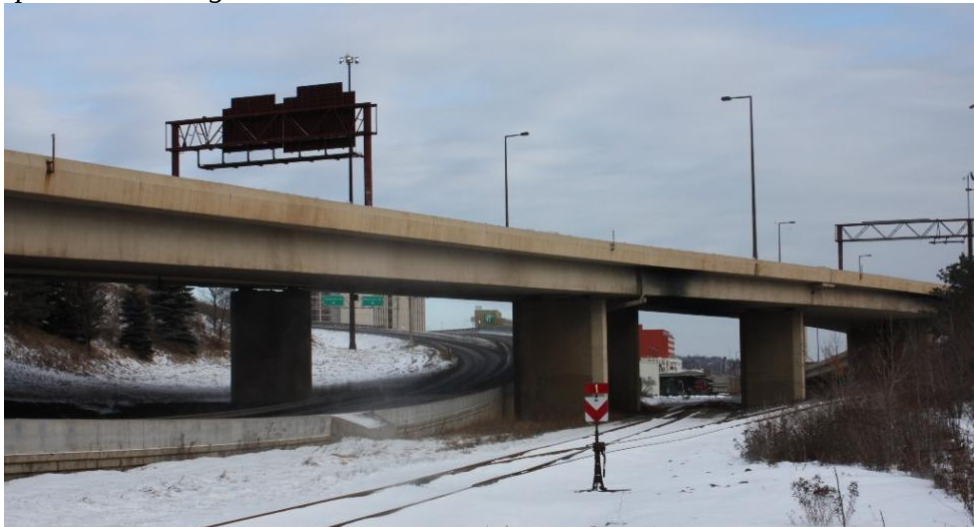
Figure 4.18. Bridge 69818 N ground view
