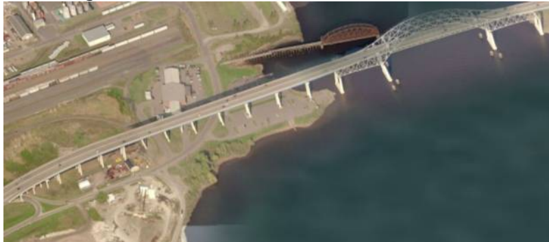
Figure 4.33. Bridge 9030 aerial view (Bing, 2011)
