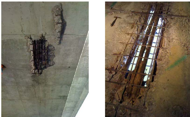
Figure 6.5. (Left) Exposed post-tensioned tendons view exterior (Corven Engineering, 2010)
