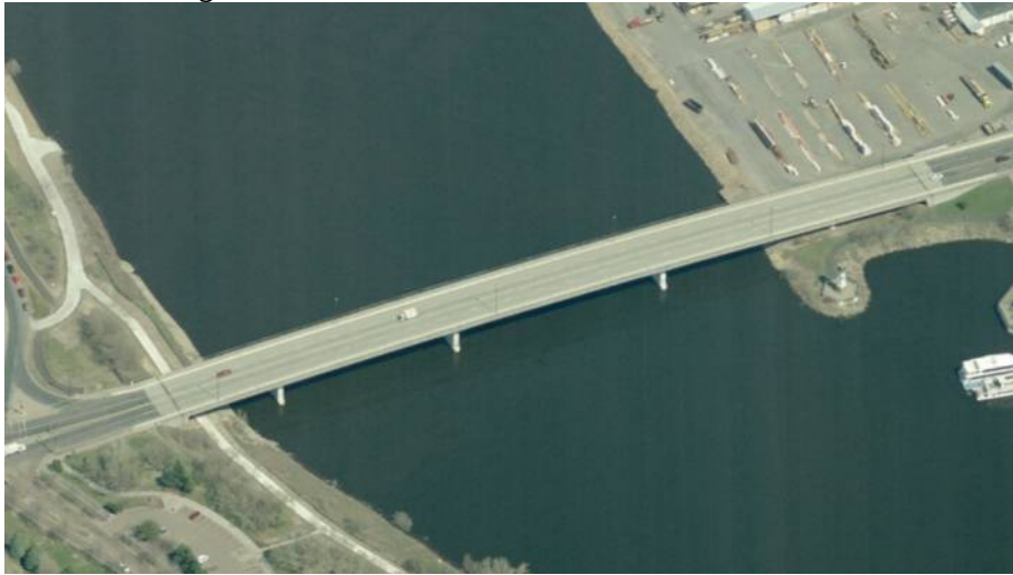
Figure 4.1. Bridge 27611 aerial view (Bing, 2011)
