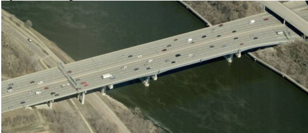
Figure 4.14. Bridge 9350 aerial view (Bing, 2011)
