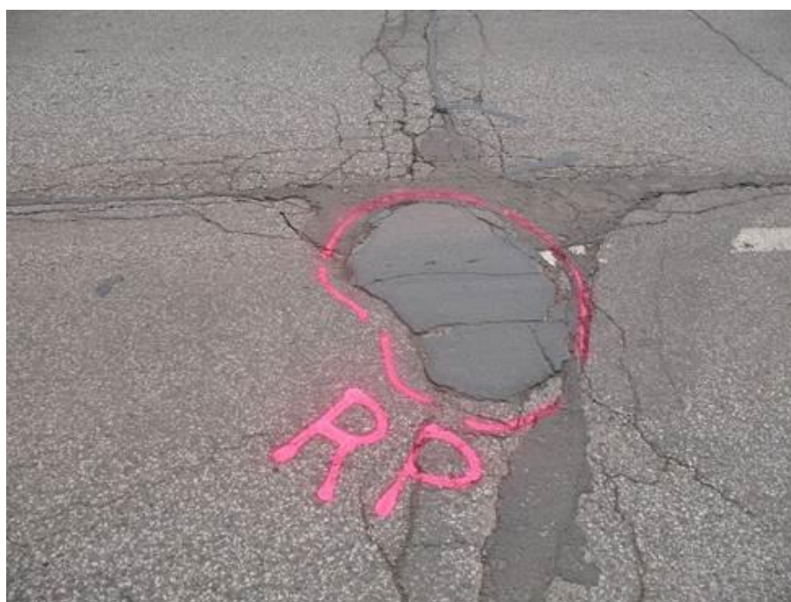
Figure 3.49. Rapid Patch repair condition, Grand Avenue driving lane: July 30, 2013.
