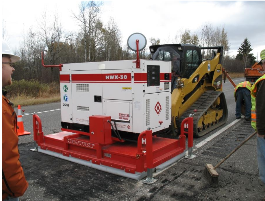
Figure 3.2. HeatWurx unit and skid-steer.
