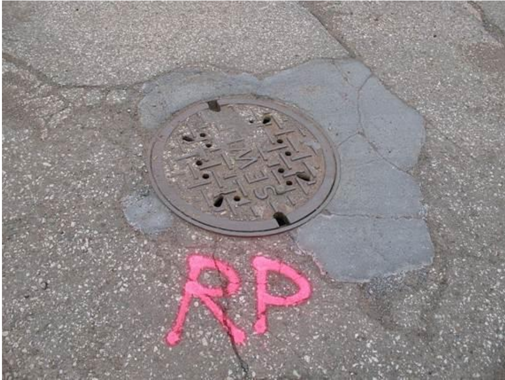
Figure 3.43. Rapid Patch manhole repair: Condition on July 30, 2013.
