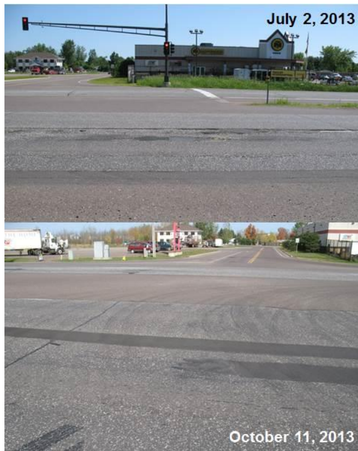
Figure 3.27. Mill-and-fill of Hwy 53/Cirrus Drive repair location.
