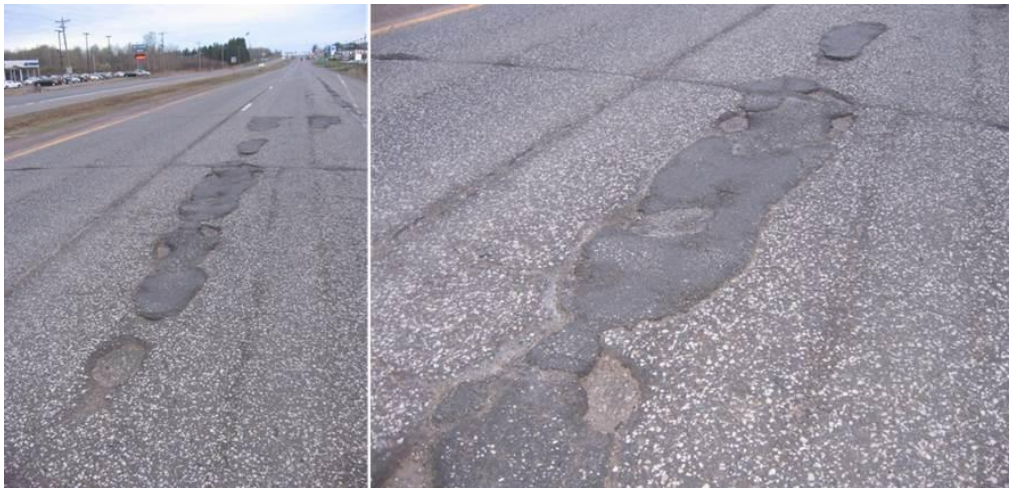
Figure 3.12. Stepp hot repair condition on May 17, 2013.
