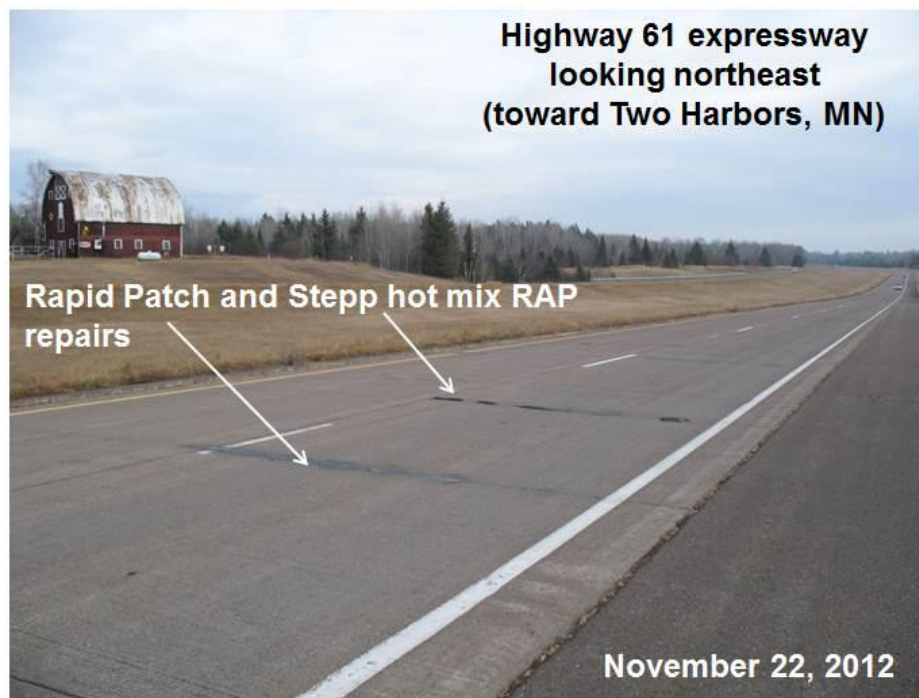
Figure 3.65. View of Highway 61 expressway Rapid Patch and Stepp hot mix RAP repairs: November 22, 2012.
