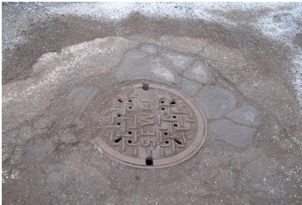
Figure 3.44. Rapid Patch manhole repair: Condition on December 26, 2014.
