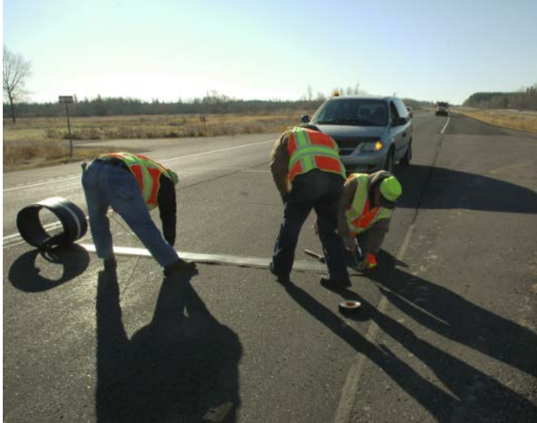
Figure 5: Weigh-pad installation at Cotton, Minnesota, TH-53
