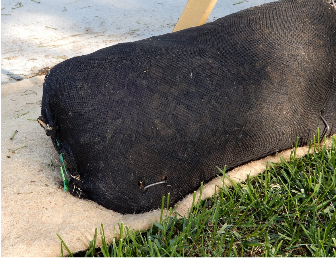
Figure 36 The end of a wood chip compost sediment control log installed using a wood fiber blanket foundation and staples placed along the leading edge. A traditional angled wood stake is also used along the downstream edge.
