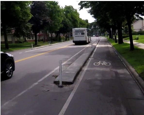
Buffer 3: Curb and Intermittent Barrier
