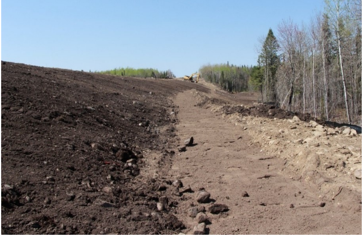
Figure 2.3 Bioslope and bioswale construction on Eagle’s Nest site in 2018.
