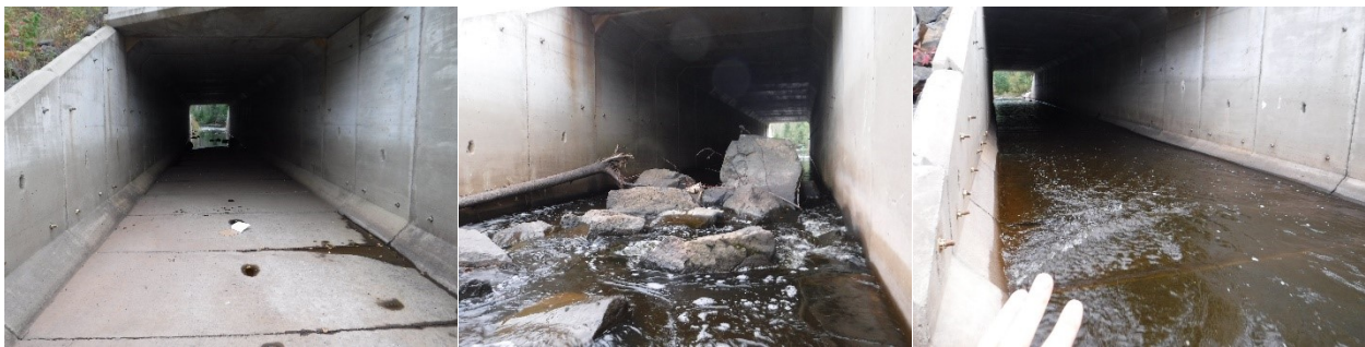
Figure 35. Photos of embedded barrel (center) and offset barrels. September 27, 2019. Barrel 1 (left) has no sediment, barrel 2 (middle) is embedded with large boulders, and barrel 3 (right) has large cobble and some boulders. Barrels 1 and 3 are vertically offset.
