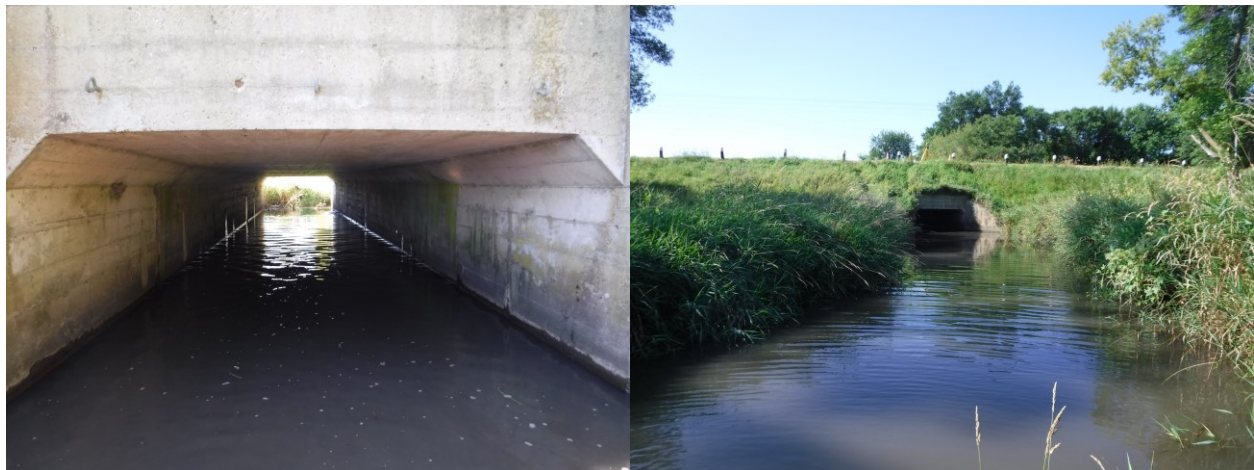
Figure 42. Unnamed tributary culvert in the Cottonwood River watershed. August 8, 2019.
