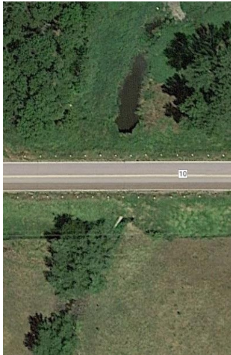
Figure 41. Aerial image of CW2. Flow is from bottom to top (South to North).
