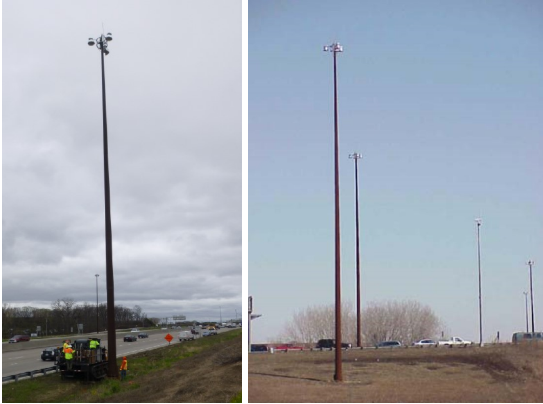
Figure 1.1 High mast light towers.
