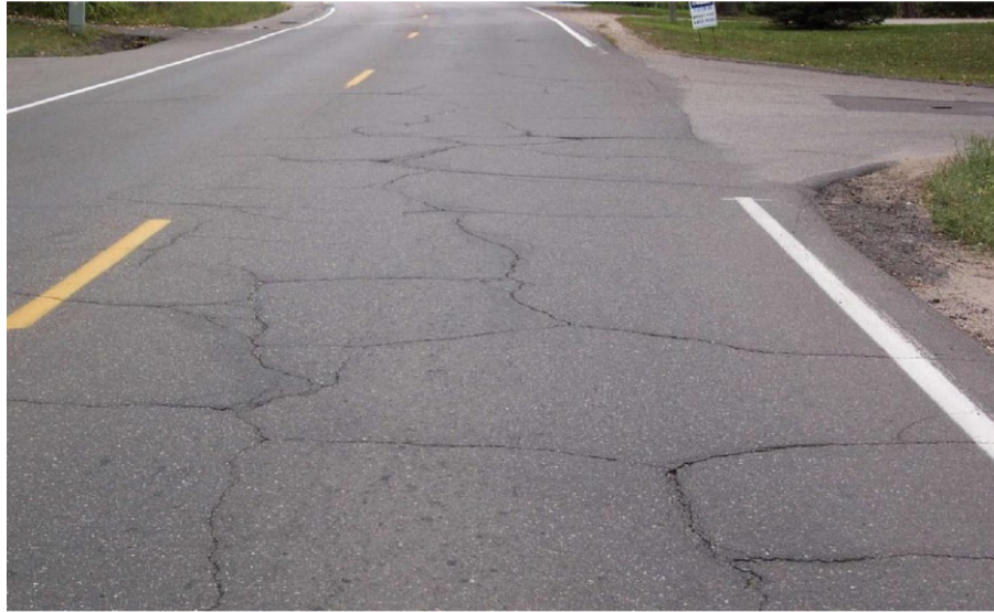
Figure A.9 Low Severity Multiple Cracking (MnDOT, 2011)
