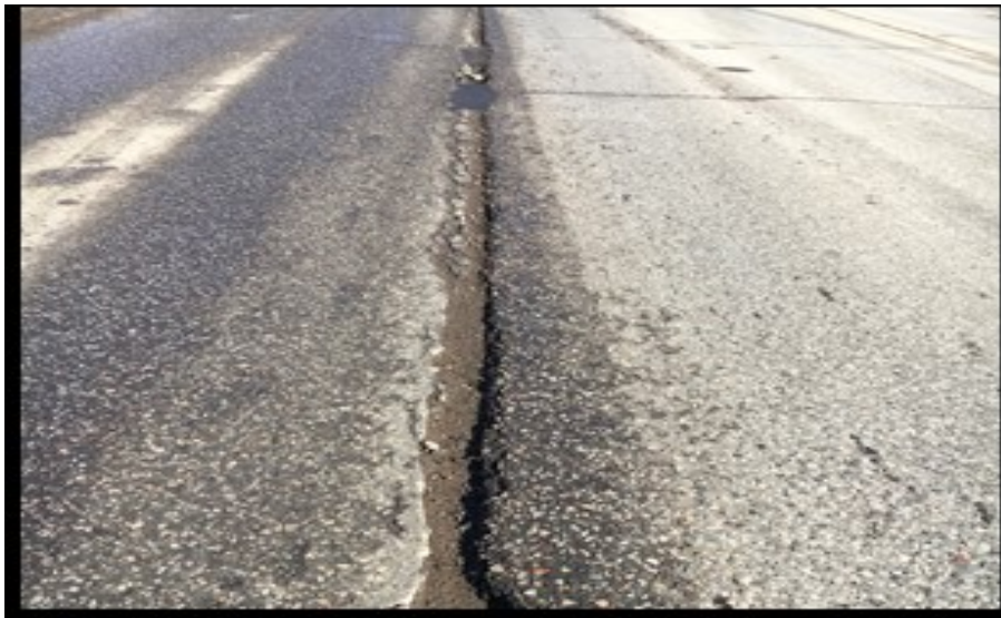
Figure A.8 High Severity Longitudinal Crack at Lane Joint (Photo Courtesy: Manik Barman)
