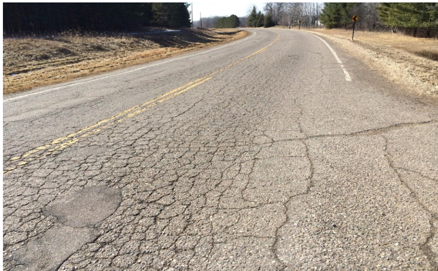
Figure A.13 Alligator/fatigue Cracking, Medium Severity (MnDOT, 2011)
