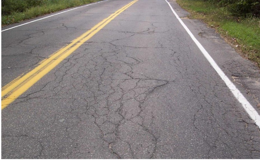
Figure A.13 Alligator/fatigue Cracking, Medium Severity (MnDOT, 2011)
