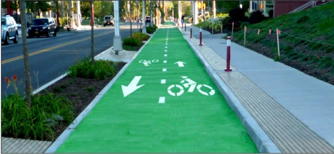
Figure 2.6 Green bike lane in NYC colored with Color-Safe™ Methyl methacrylate (MMA) (Grossman, 2017)
