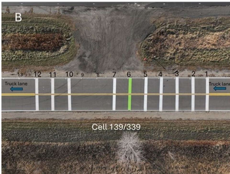
Figure 5.4 Drone view of Cell 46 (A) and Cell 139/339 (B) pavement markings
