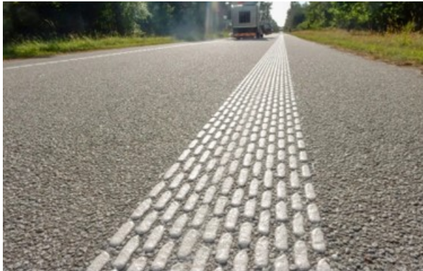
Figure 4.19 Geveko Markings new road marking profile (Geveko, 2018)
