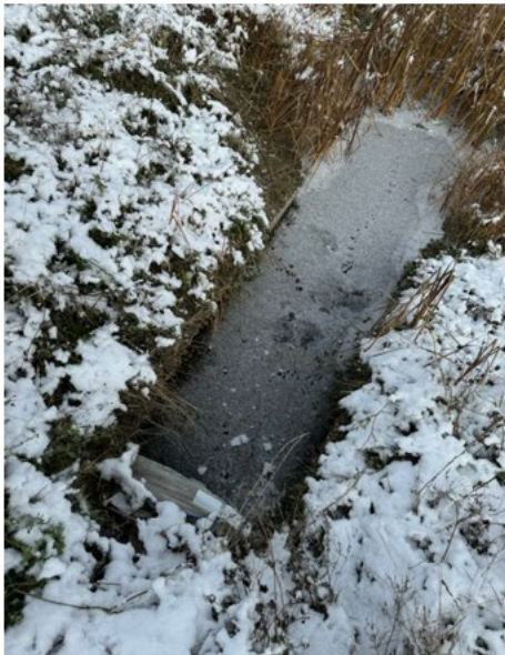
Figure 3.11 Inspection; 2 in. of ice was estimated, and the culverts were not accessible
