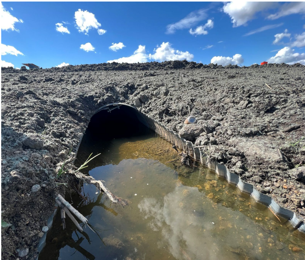
Figure 2.24 Photograph of culvert taken 30 days after installation
