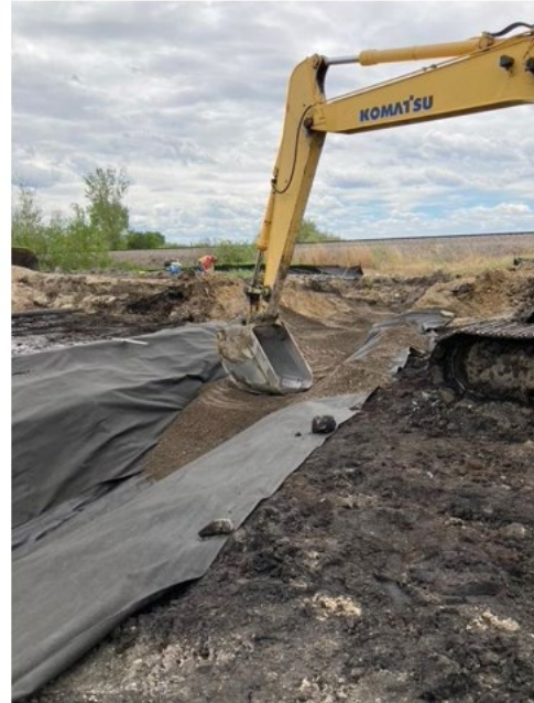
Figure 2.9 Wrapping the trench in geotextile to prevent mitigation of fines into backfill
