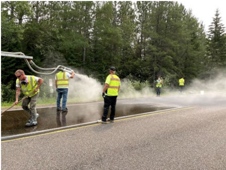
Figure 6.5. Dust monitoring by industrial hygienist downwind of HFST aggregate deployment
